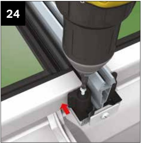
24 Centralise the glazing between the glazing bars. If necessary pack it out on each side - press it down onto the support trim. Using the fixings provided, screw down into the bar as shown.
