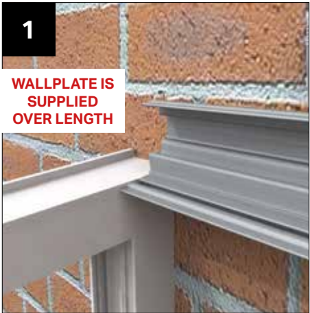
Offer the wallplate up to the wall and position it so that the top surface of the bolt slot is level with the top of the side frames.
