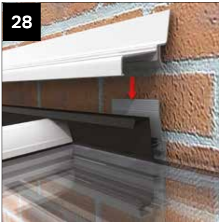
28 Cut the PVCu wall plate top capping to the overall width of the conservatory (externally) and notch over the top of the lean-to cloaking trim at each end. Push fit the wall plate top capping.
