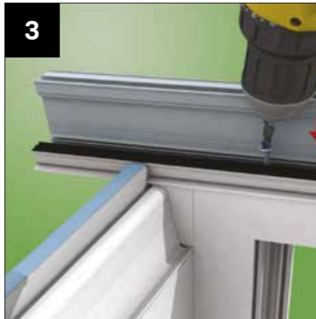
Screw fix the glazing bar down into the head of the raked frame at 500mm centres. Continue to fit the glazing as in steps 20-23 in main guide.
