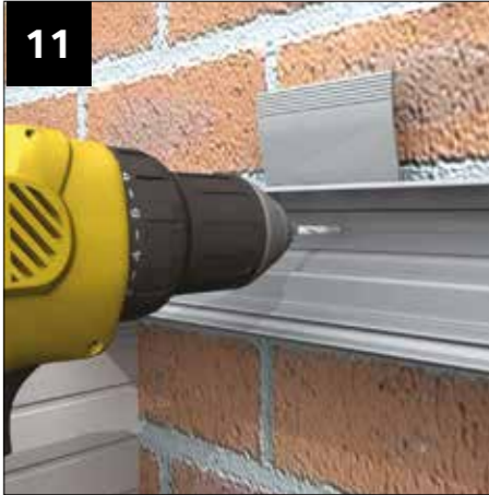
Drill through the wallplate main body and directly through each carriage to suit the masonry anchors being used (not supplied). Mark the position of each masonry anchor on the house wall and drill the house wall to suit.
