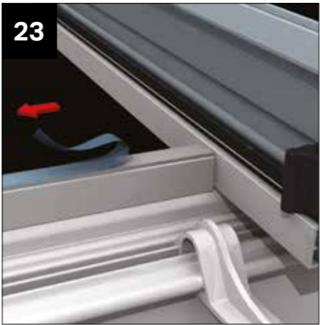
23 Tease the 'tail' of the glazing support trim tape free (ready to be pulled away when the sealed unit is finally in position).
