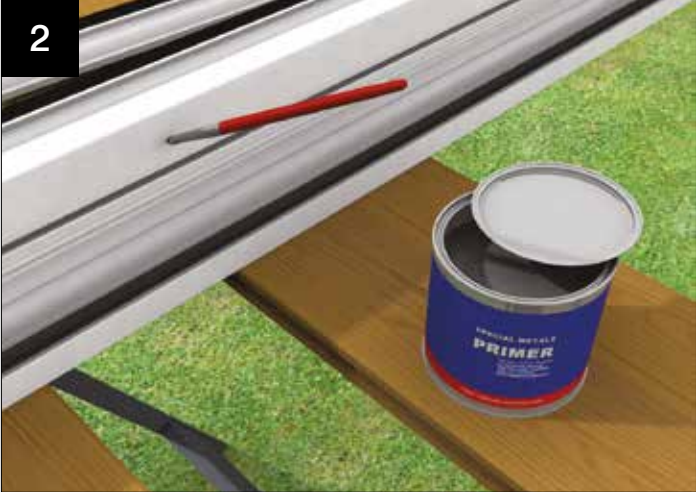
Ensure the surface is dry – apply a thin primer coat using a fine brush.
