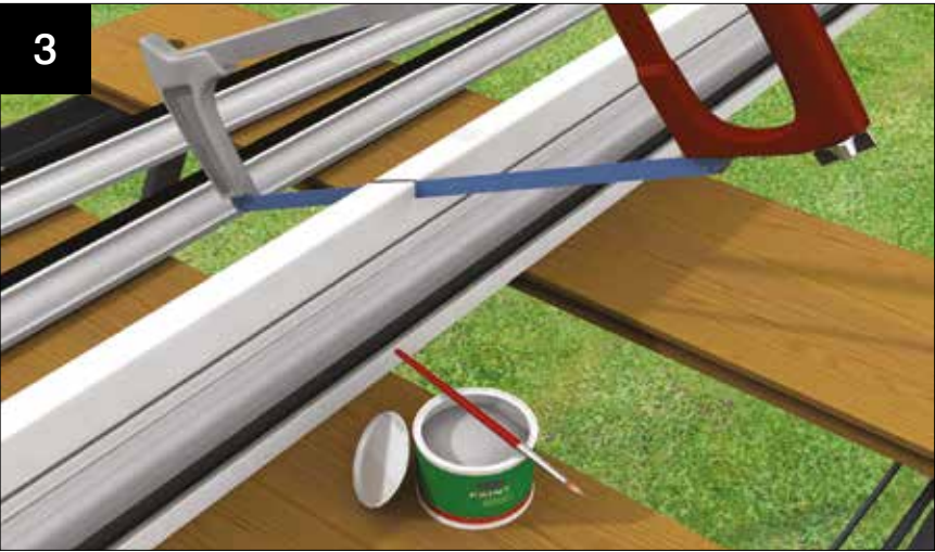
If site cutting is necessary (drainage slots need inserting or a down pipe hole has to be cut) ensure all swarf is kept away from the painted surface and then seal with a primer/corrosion inhibitor and then top coat. Alternatively, use a suitable gap sealant to prevent the onset of corrosion. These steps are critical in marine environments.
