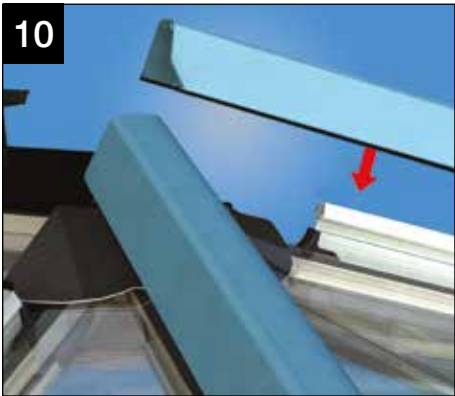
Install bar caps, securing flashing into place. Point around bar caps.
